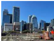
(Convention Center建設現場)
