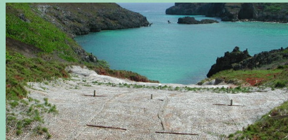
Situation after installation of topsoil conservation sheet (2002)
